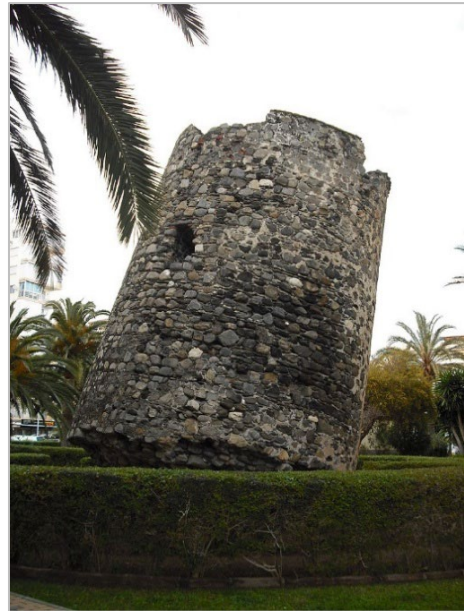
Fig. 8- Torre Ladeada in the town of Algarrobo (WikipediaCommons, JSpain).
