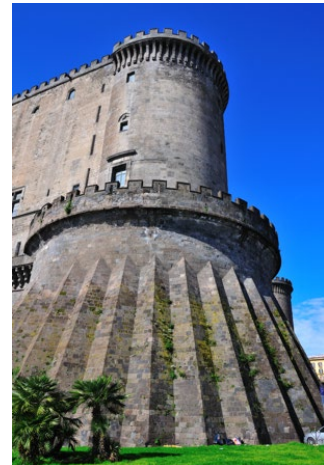
Fig. 14- A view of a port turret with anti-artillery reinforcement and ricochet device. Source: https://historiemedievali.blogspot.com/2017/04/castel-nuovo.html
