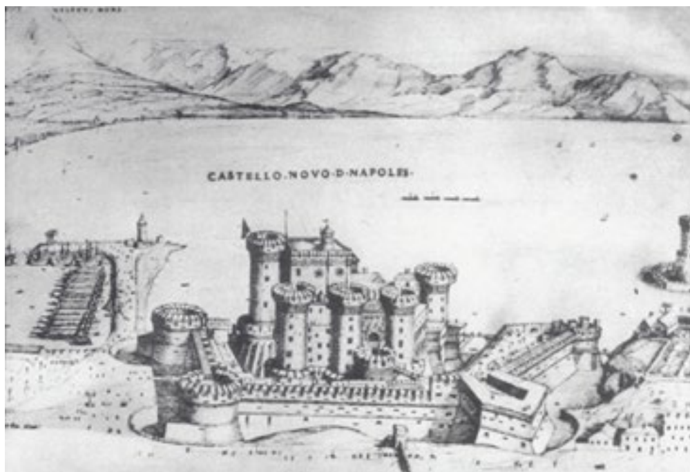
Fig. 15 – Castello Novo D Napoles - The Castle opens onto the Bay of Naples with its military port (on the left: the city's fleet of galleys), providing protection with a double fortified ditch, with the external protection dominated by an impressive low wall with devices for artillery, and a pentagonal bulwark in counterpoint with the solution of cylindrical turrets and bastions (Holanda, c. 1540, f. 53v).
