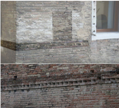
Fig. 11- Venice: the round corner and the traces of a demolished frame belong to a previous crenellated wall close to the Prigioni Nuove (Angela Squassina, 2024).
