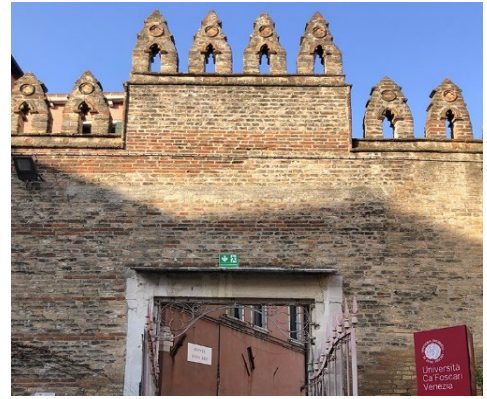
Fig. 9- Venice, Ca Foscari: a fine manufactured version of late gothic three-foiled brick merlons (Angela Squassina, 2024).
