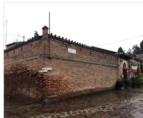
Fig. 7- Venice, Giudecca: the simple saw-shaped crenellation of the front entrance wall of Officine Navali Toffolo in Giudecca (Angela Squassina, 2024).
