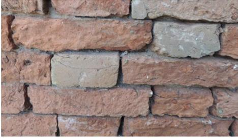
Fig. 15- Erosion of mortar joints, San Rocco fort (photo by Fabio Fratini, 2024).
