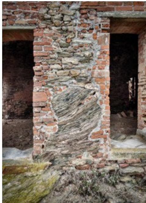
Fig. 4- Stone from the cliff merged into the masonry work at the upper base of the tower (photo by the authors, 2024).
