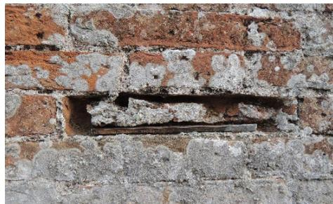
Fig. 14- Brick erosion and biological growth, San Rocco fort (photo by Fabio Fratini, 2024)
