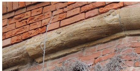
Fig. 10- Stringcourse in Pietra Panchina, Bibbona fort. Exfoliation phenomena in ashlar laid with the layering parallel to the surface of the masonry (photo by Fabio Fratini, 2024).
