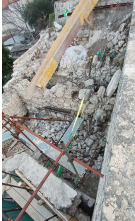
Fig. 9- The pulling of the western wall (Fortress of Culture, 2022)
