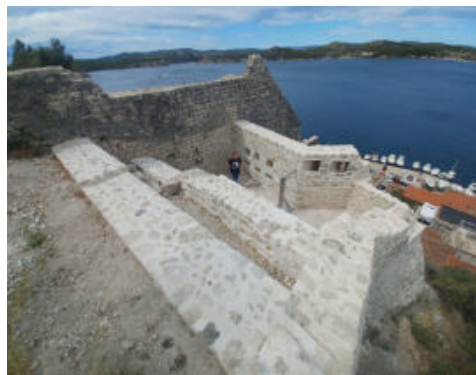
Fig. 10- Sperone after the completion of construction works (Fortress of Culture, 2022)
