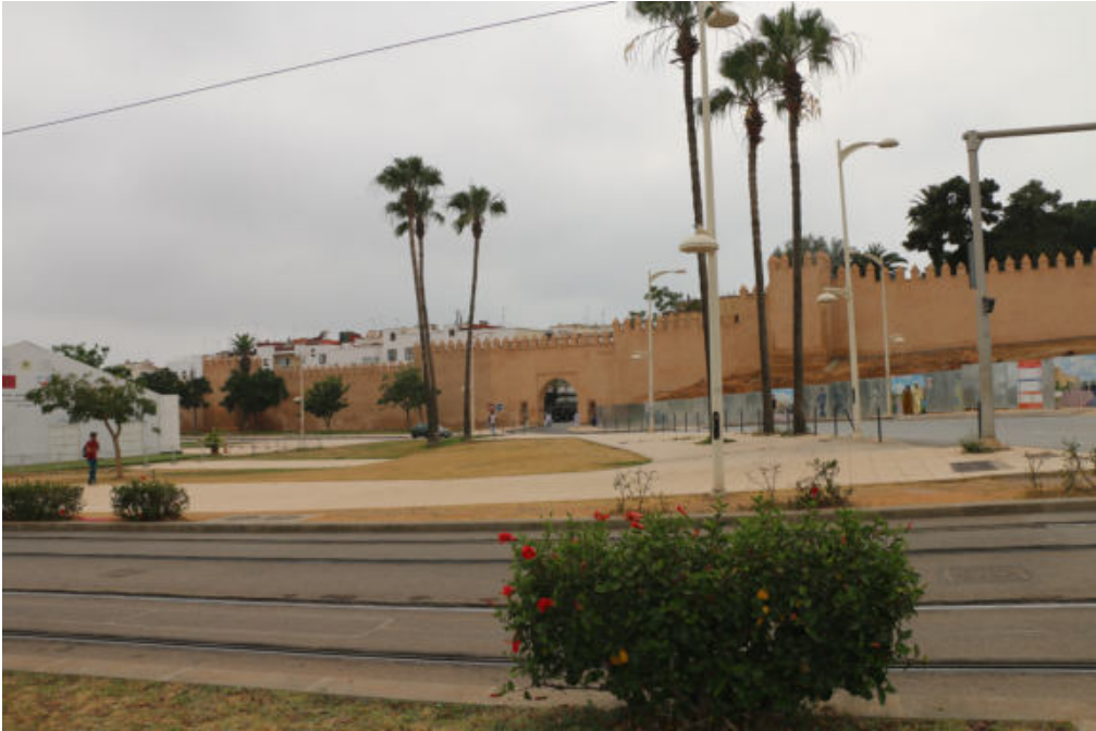
Fig. 4- Houses in the new Mellah (the new Jewish district) next to the wall where was the port and orchards (photo by Magyda Cherradi, 2022)
