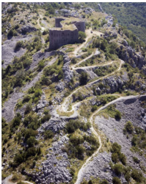
Fig. 9- Serpentine approach road to Fort Kosmač (photo by Radojica Pavićević, 2010)
