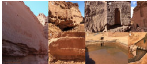
Fig. 4- Tafza constructive know-how of Taouehsit Tafza mâallems , limestone master-builders (photos by author, 2019)
