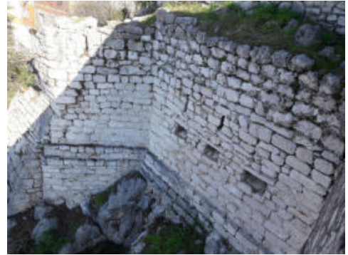
Fig. 5- Arrowslits and firearm openings on the western wall (Fortress of Culture, 2018)
