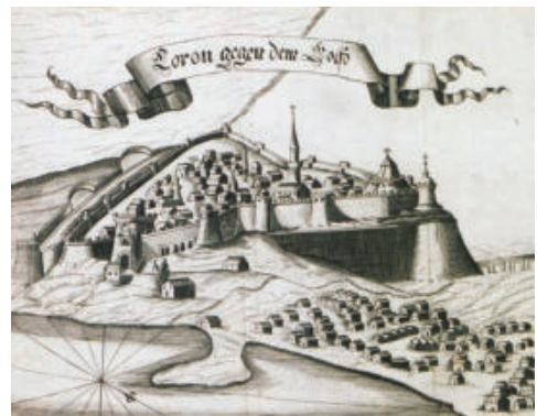
Fig. 5- The multi-storied ottoman tower and the outermost tower-bastion and semi-bastion are depicted in the plan Coron gegen dem Golfo (Enderlin, 1686, travelogues.gr)
