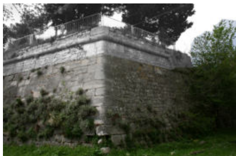
Fig. 10- Traces of tenaglia (from construction stage 1) in construction stage 4 - in colour (photo by Snježana Perojević)
