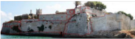
Fig. 7- Stratigraphic survey of the north wall of the castle (D'Amico, 2017)
